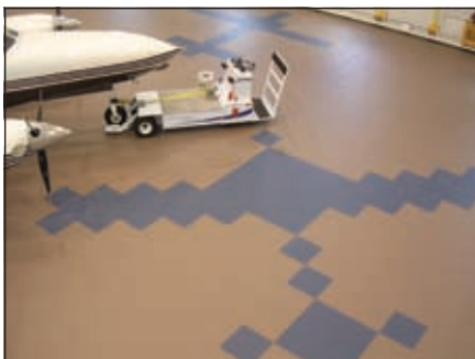
SwissTrax, top, is popular for trade booth floors. Tuff-Seal joins with dovetail joints, second from top, while SwissTrax uses a hook and eye arrangement. For large hangars, patterns can indicate aircraft placement.
